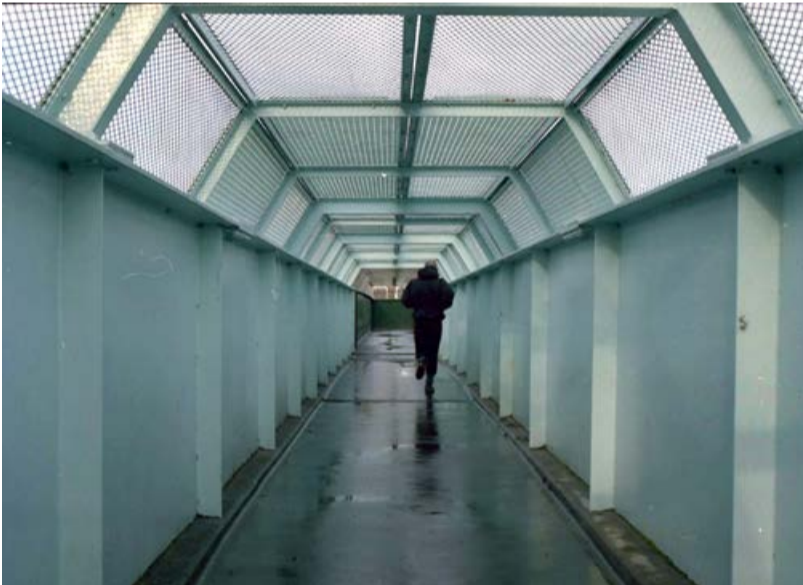
Caged bridge to be avoided
