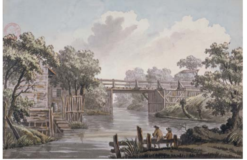
Historic Timber Bridge
