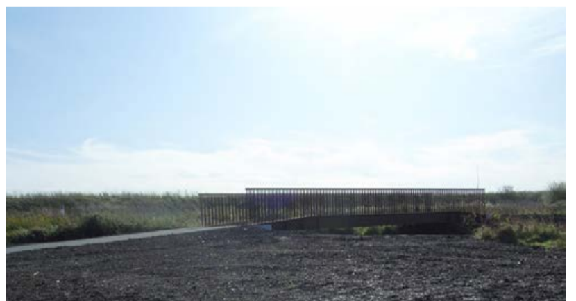
Steel Bridge, Rainham Marsh
