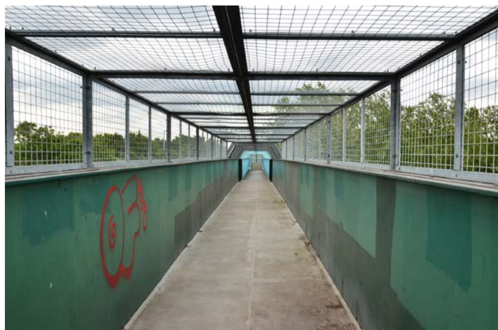
Carbuncle Bridge looking east towards the marshes
