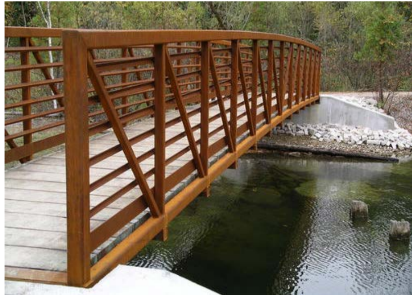
Corten Steel Bridge
